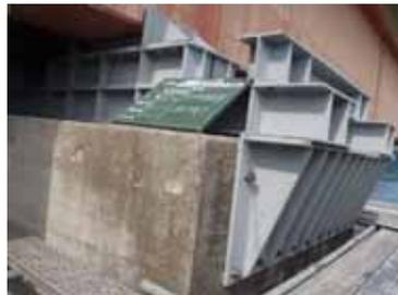
Photo 8 : Temporary repair work for bearing
